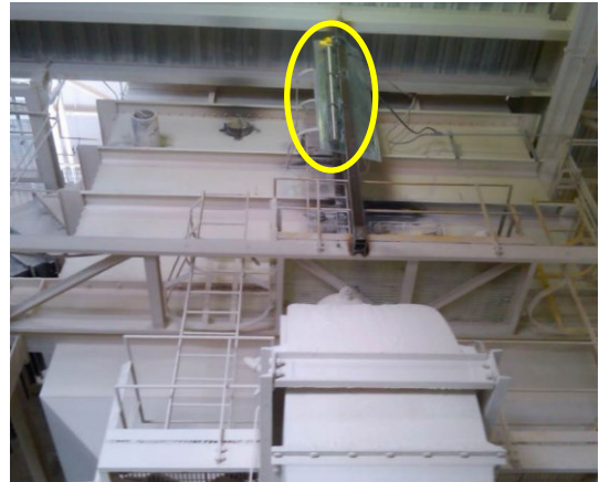
Figure 2 - The upper ambient temperature limit for radiometric detectors is about 150°F.
