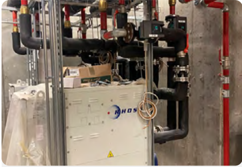
Installation of a heat pump at VEGA Italy
