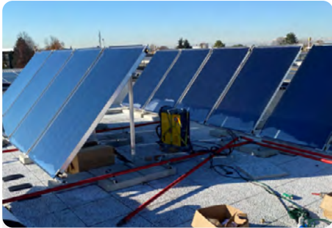
Photovoltaic system at VEGA Italy
