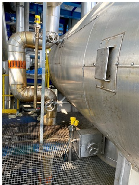
VEGAFLEX 81 guided wave radar sensors measure the separation layers in the 3-phase separator.
