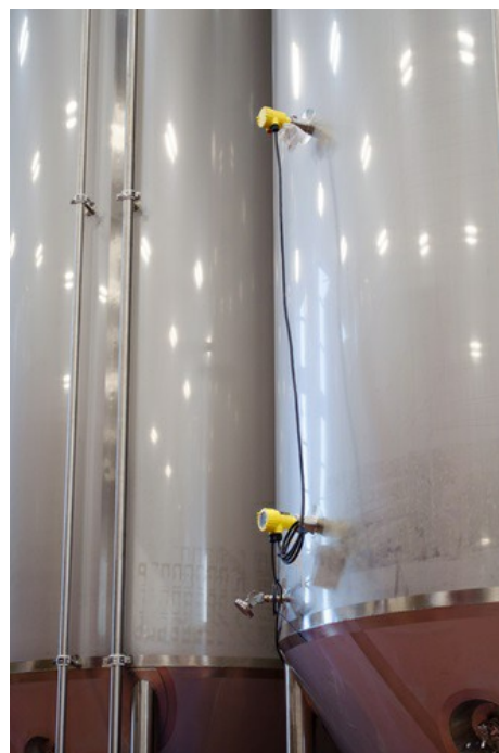
Two VEGABAR pressure transmitters connected by a cable are installed on the vessel – one near the bottom and another near the top.
