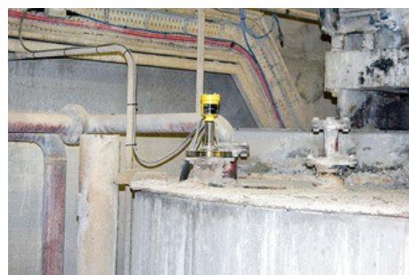
VEGA 80 GHz radar level sensor installed very close to the edge of the milk of lime mixing vessel.
