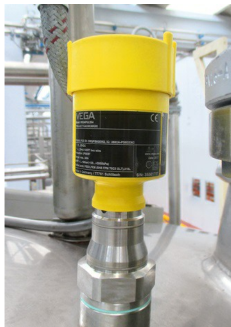
VEGAPULS 64 measures reliably even when faced with viscous build up, in this case chocolate, and difficult installation situations, e.g. caused by agitators.
