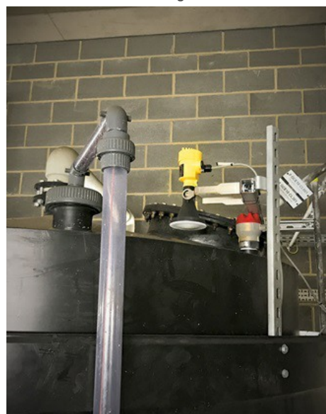
A VEGAPULS 64 radar sensor, mounted above a storage tank on a boom, measures the level of hydrochloric acid right through the top of the tank.
