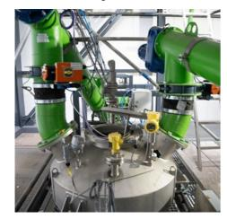
The measuring instruments are positioned along the entire recycling process, ensuring efficient workflows within the various operational steps. They can also be found in the reactor, at the heart of the whole processing facility, which Pyrum holds several international patents on. There, VEGA measuring instruments monitor and diagnose the reactions and make sure that they are taking place within the prescribed limit levels and pressure ranges.
