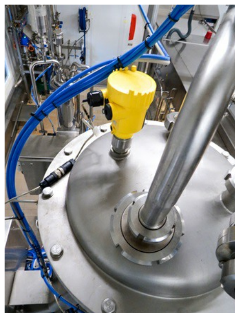
VEGA sensors control the level to keep the yoghurt filling process running smoothly.
