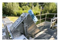
The radar sensor provides an exact overview of the levels at multiple points in the sewage treatment plant.
