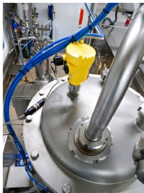
VEGA sensors control the level to keep the yogurt filling process running smoothly.
