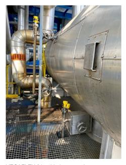
In a 3-phase separator, the VEGAFLEX 81, a level sensor based on the guided wave radar priciple, can measure the hydrocarbon/water interface. The data is necessary for controlling the amount of water that is pumped from the container to the wastewater treatment plant. This prevents the unwanted escape of hydrocarbons. Continuous level measurement in the floors of the column is necessary.
