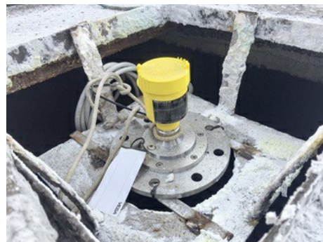
Salt deposits made life difficult for previous sensors.
