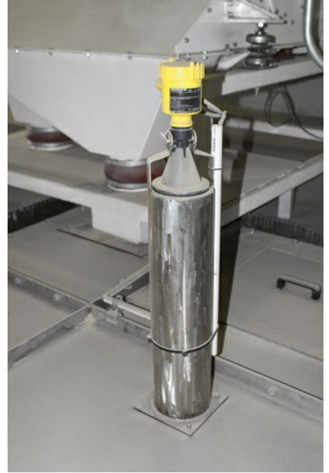
Despite the significantly shorter wavelength of VEGAPULS 69, the sensor is very insensitive to deposits.
